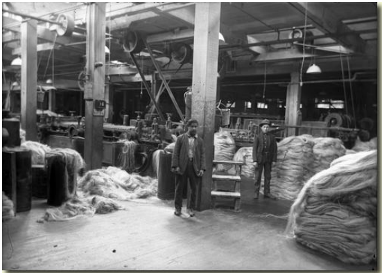
Hemp Processing Machine Room Submitted by A. Storm
